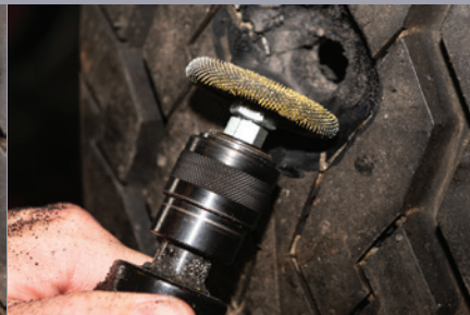
Use a Medium-Grit Rasp to Texturize Repair Area
